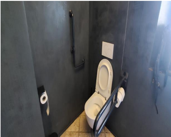
27 Toilets and grab bars
